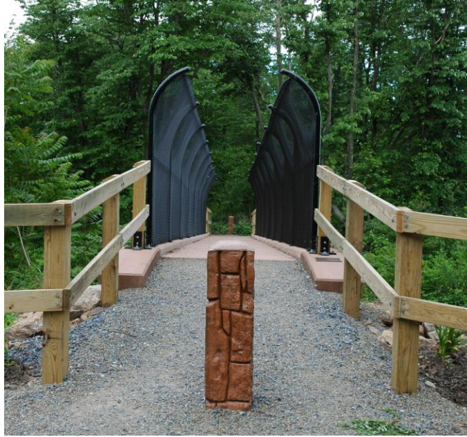
Bridge over Rt.225 5/30/2004 (Peter's Mt. 10 photos)
